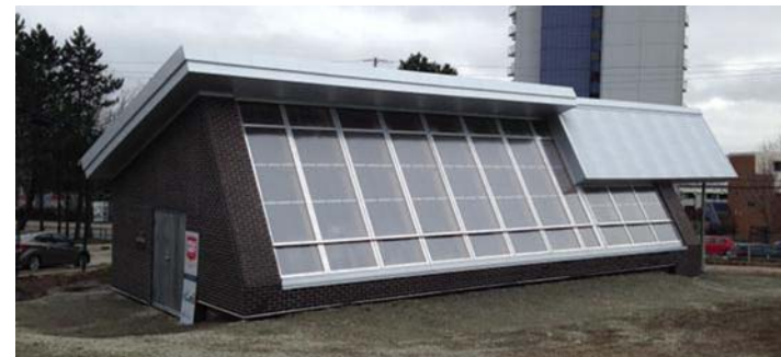
Hope Blooms' state-of-the-art greenhouse was built along with our contractors under the Build Right Nova Scotia initiative (a cooperative of contractors and the 11,000 tradespeople that make up the Building Trades).
